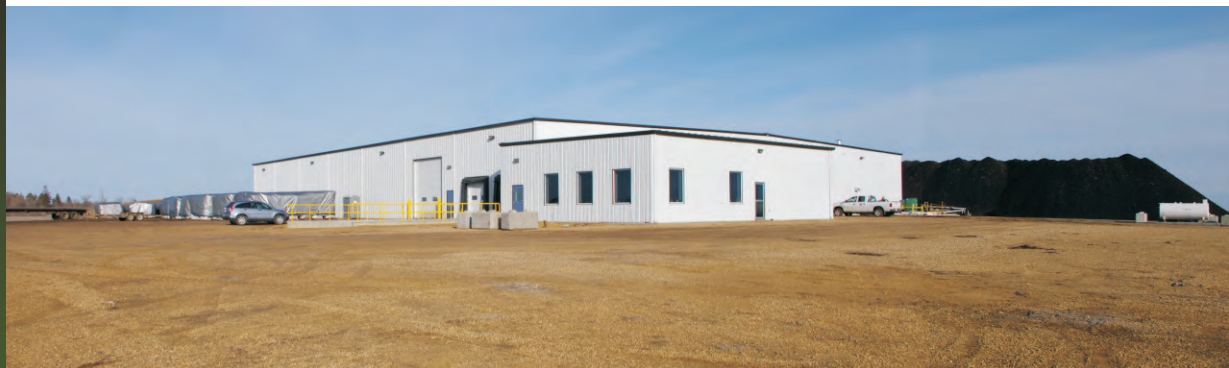
Black Earth Humic Production Facility in Ryley Alberta, Canada
